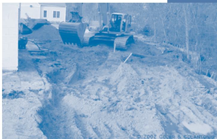
Excavation down to bedrock layer
