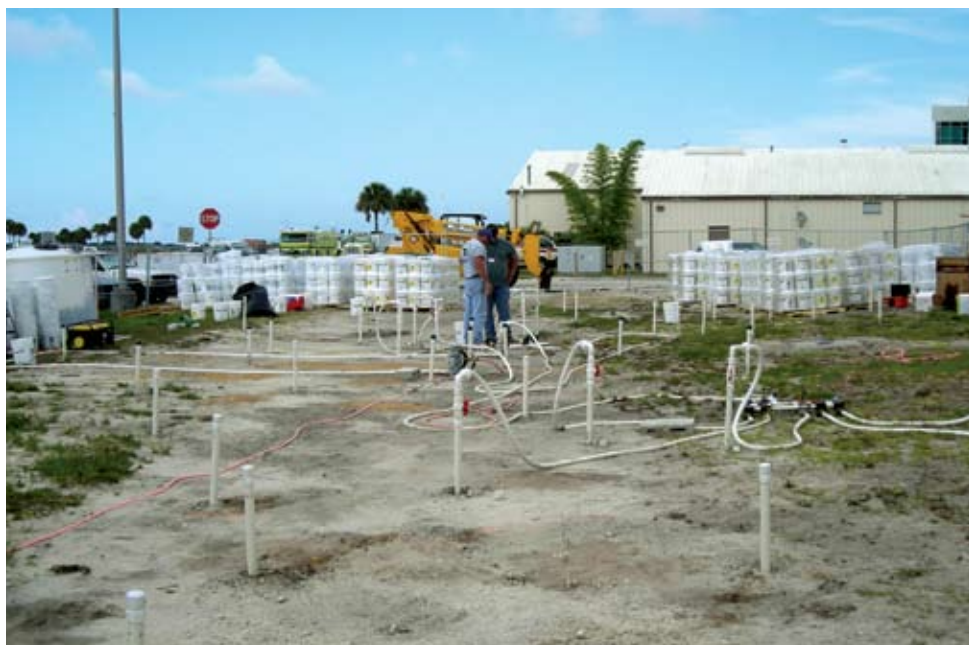
A total of nine injection events over 10 months reduced the remediation costs by about 75 percent.
